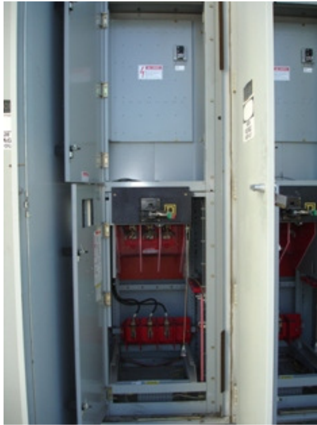
MCC-03 Future 350HP Pump Starter Interior Elevation
